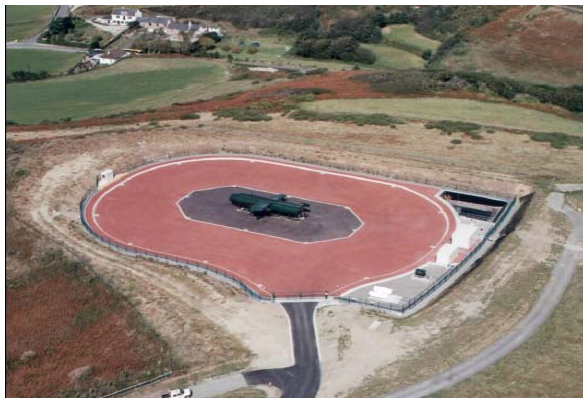
Aerial View of new Fire Training Ground
