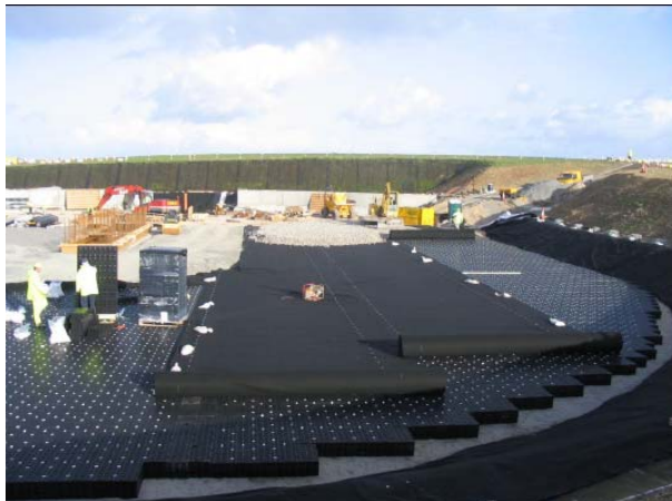
Construction of the below pavement storage cell
